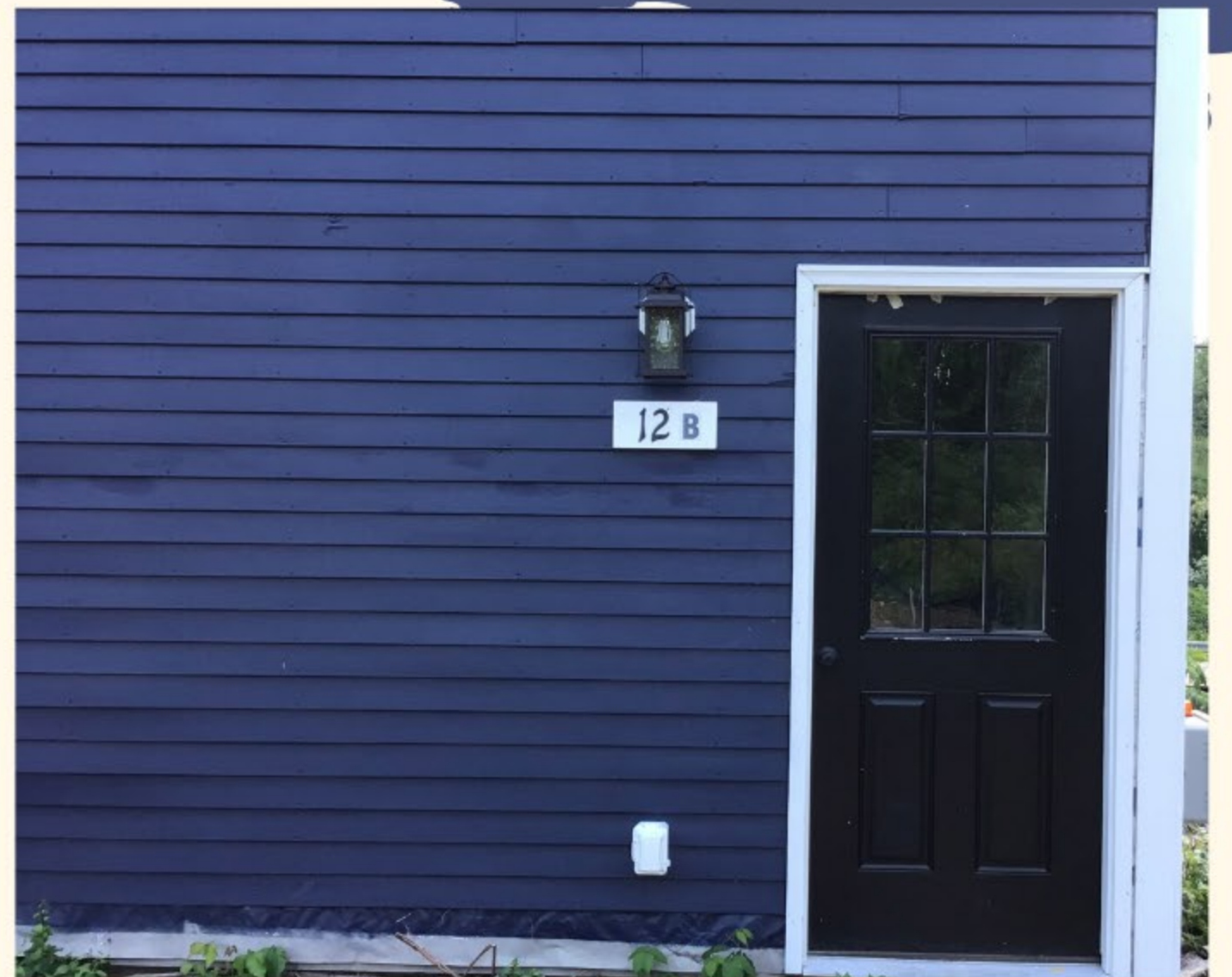
View of Back Door
